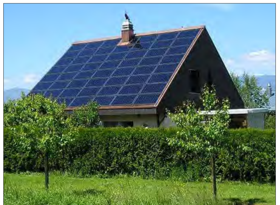
An example of how on-site renewable power generation such as photovoltaics can be integrated into the massing of a building.
