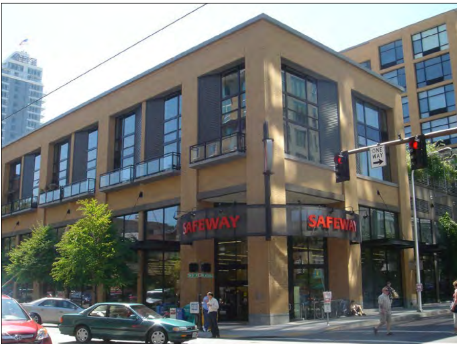
A mixed-use building with direct access into ground-floor commercial uses through shopfront frontages on both street facades.
