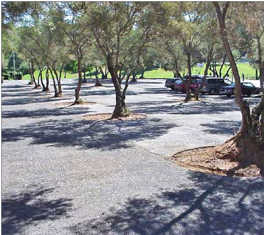
Permeable paving allows stormwater to percolate and infiltrate through areas that are traditionally impervious, such as large parking lots.
