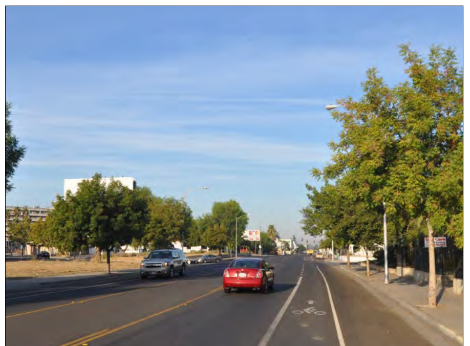
Divisadero Street re-striped as a 3-lane street with bike lanes and parking on both sides.
