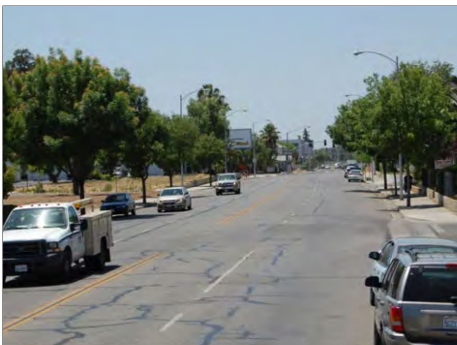
Divisadero Street as a wide 4-lane street with parking on both sides.
