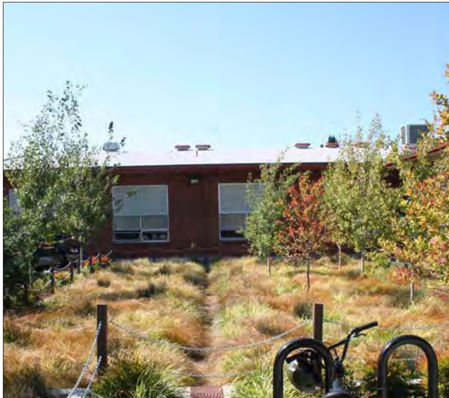
Rain gardens – planted depressions to capture rainwater runoff – allow stormwater to soak into the ground locally instead of flowing into storm drains.
