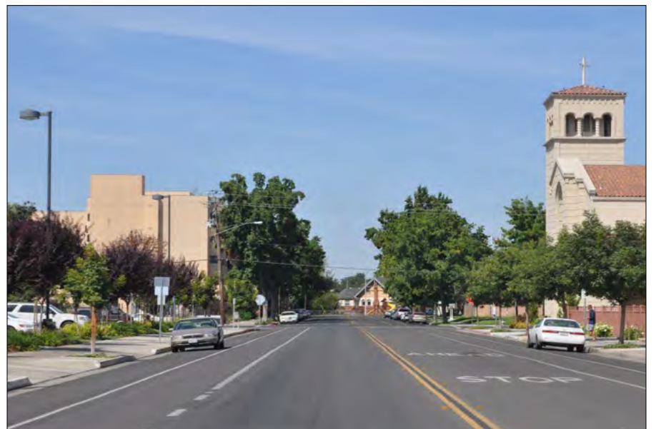
View of M Street near Stanislaus Street with a road diet.
