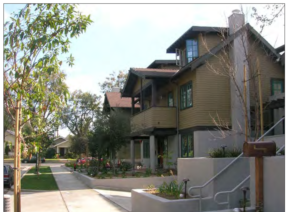
A new building (at right) fits into a single-family Craftsman era residential neighborhood by providing compatible massing and porch frontages.
