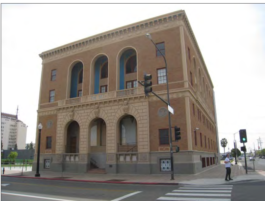
The Fresno Bee Building (1922) on Van Ness Avenue was adaptively reused as a broadcast studio and office space.
