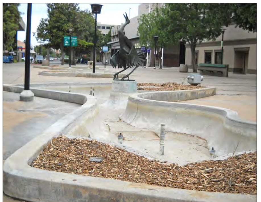
Leaky and empty fountains and missing irrigation gave the Mall an abandoned look.
