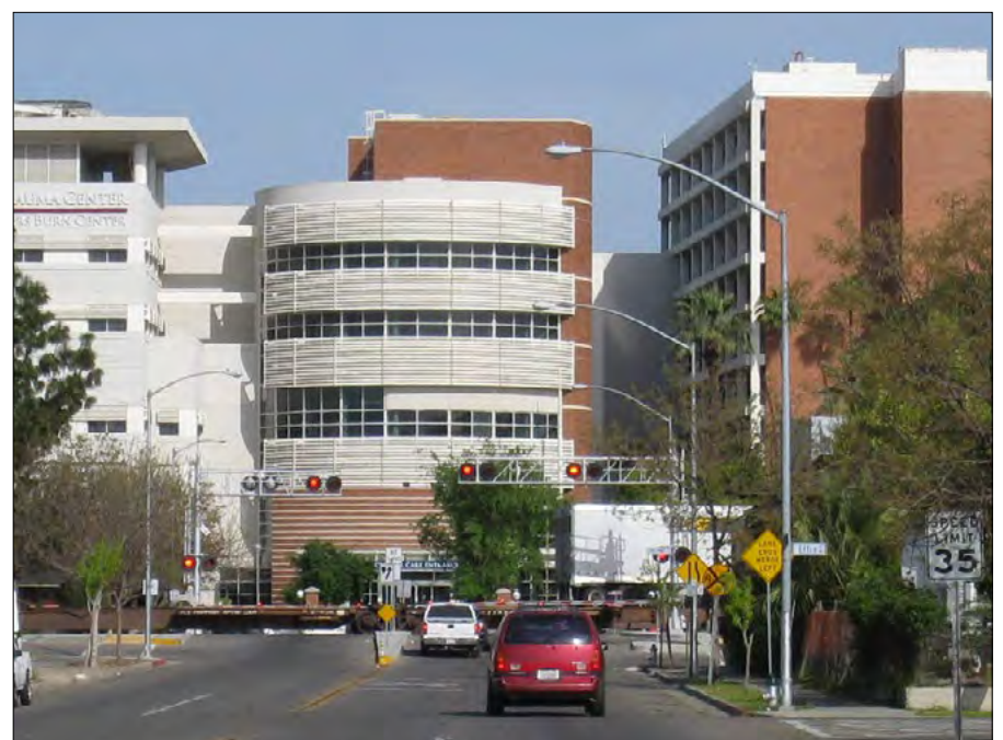
View of the Divisadero Street at-grade BNSF railroad crossing and Community Regional Medical Center.
