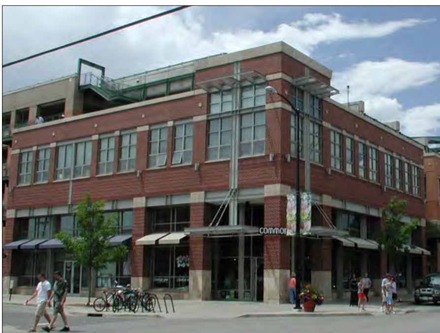
This park-once garage is hidden from the view of the street by occupied uses: retail on the ground floor with upper floor offices.
