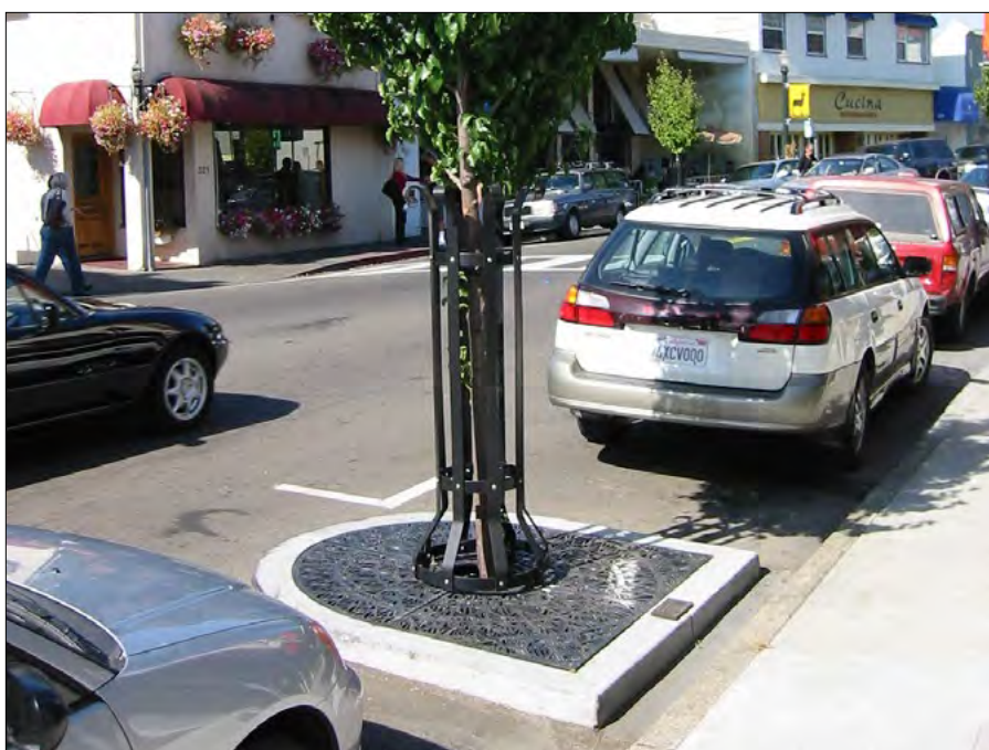
In-street bulb-out brings the trees closer to the automobile traffic to narrow the perceived width of the street while allowing an uninterrupted pedestrian path on the sidewalk.
