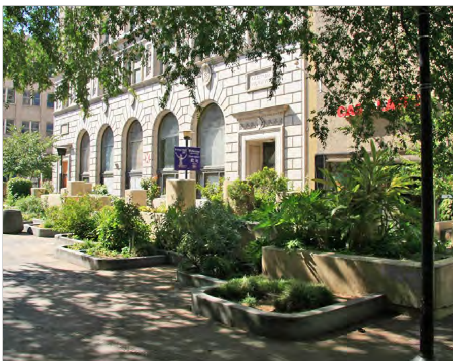
The overgrown foliage in a planter that used to be a fountain blocks views into storefronts.
