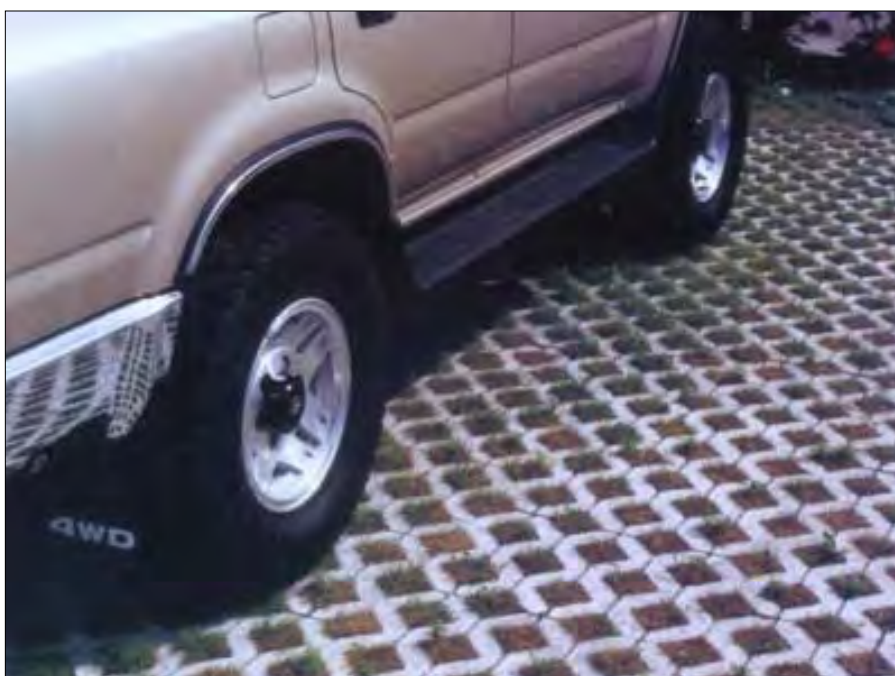
Pervious paving within parking areas provides on-site stormwater infiltration and reduces runoff.
