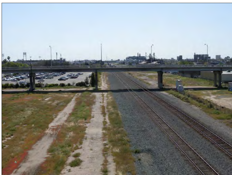
View of the grade-separated UP railroad crossing at Tuolumne Street. CHSRA will remove the Stanislaus Street Bridge and widen the Tuolumne Street bridge to accommodate two-way traffic.
