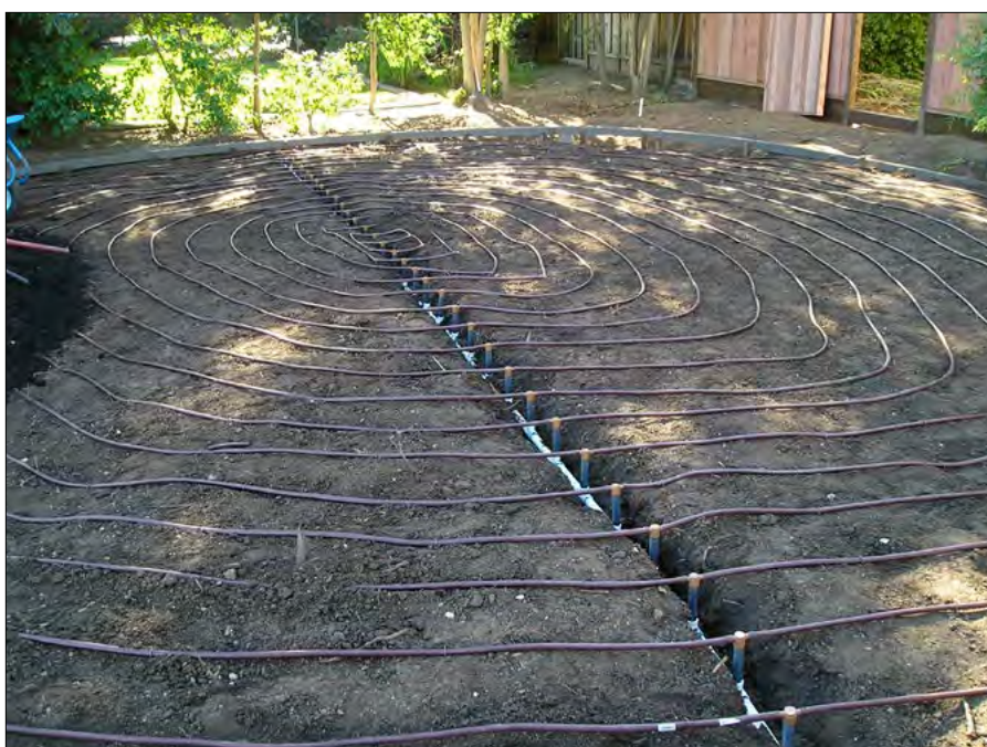
Drip irrigation allows water to drip slowly to roots and reduces the amount of water otherwise lost to evaporation in a typical sprinkler system.
