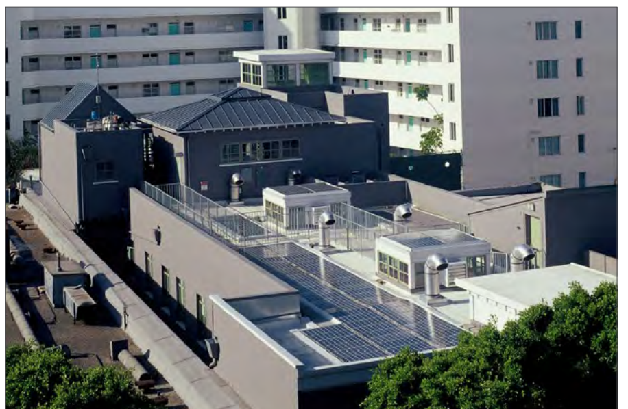
An office building utilizes rooftop solar panels and natural light and ventilation from rooftop light monitors.
