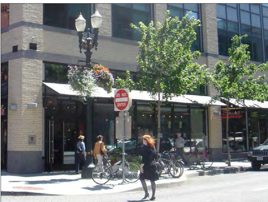
A mixed-use building provides transparent storefronts and awnings over the sidewalk to provide an enticing and comfortable environment for pedestrians.
