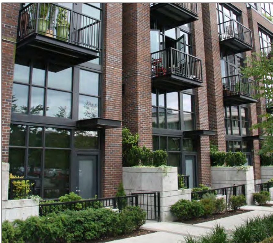
Ground floor Live/Work units with patios and entrances set back from the sidewalk. Upper floor flats and townhouses have balconies facing the public realm.
